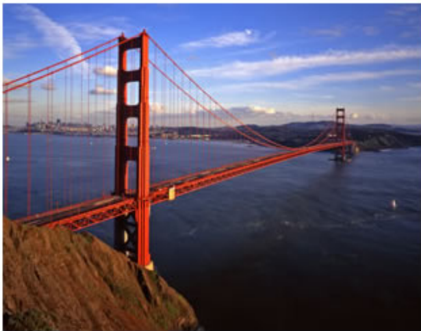
Golden Gate Bridge, San Francisco
